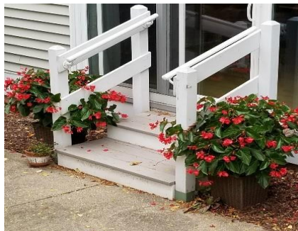
#5 ACCEPTABLE Two handrails
