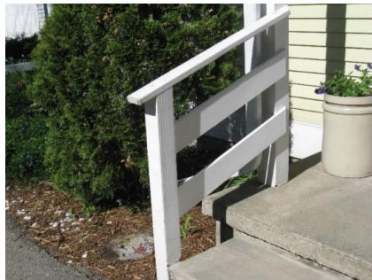
#2 ACCEPTABLE Graspable handrail
